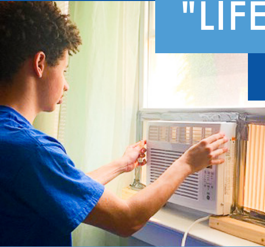
ElderCool Intern John installs an AC unit.
